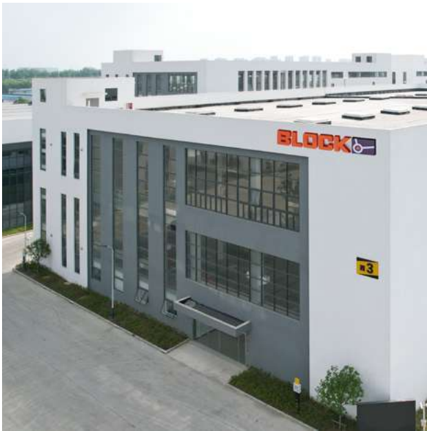
Usine Kunshan, Chine Factory Kunshan, China
